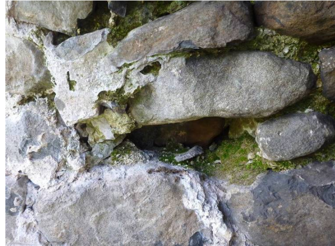
Fig 21 Socket from which stone fallen out in arch
