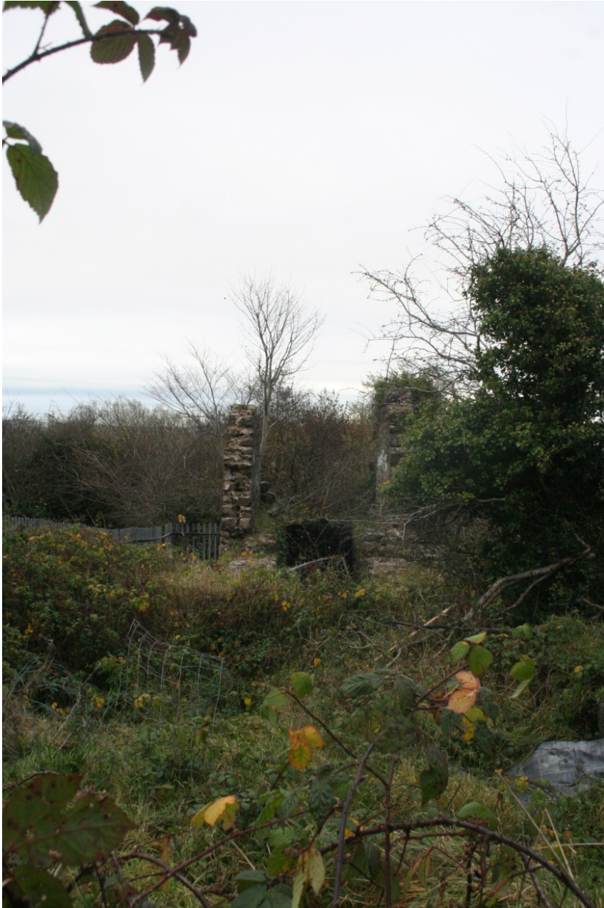
Figure 6.2 – The overgrown remains of the wheel pit, looking east.
