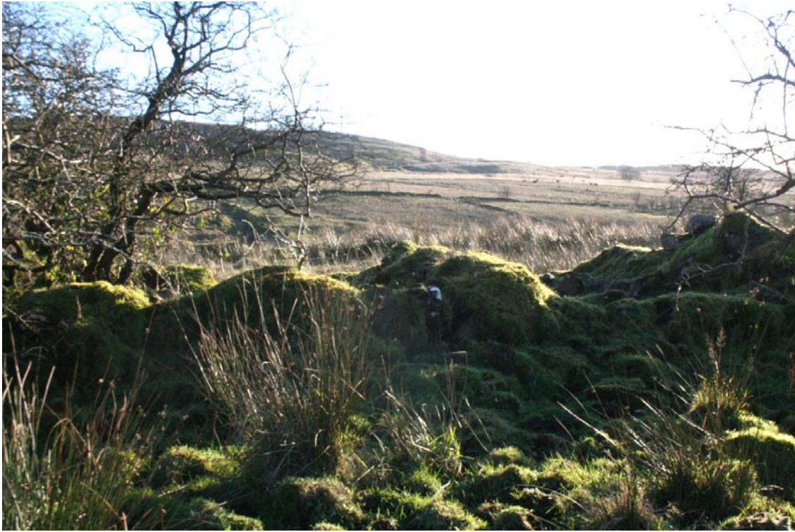
Figure 12.6 – Grass and moss covered remains of the row of buildings, looking south-south-west.
