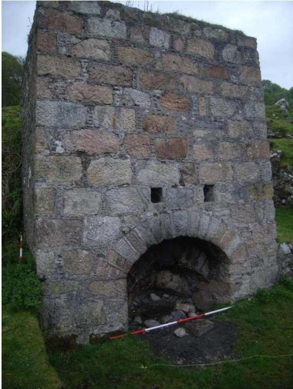
Figure 2.10 - Lime kiln, Muroolough Bay, Co. Antrim (from Welsh 2011, figure 2).
