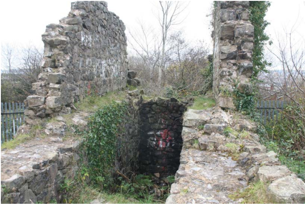
Figure 6.3 – The wheel pit, looking east.
