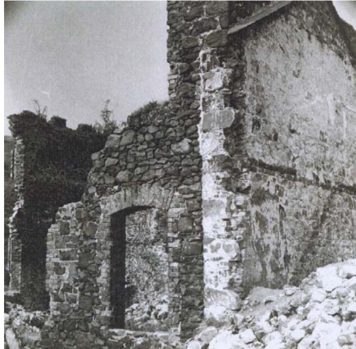
Figure 4.7 – The mill gable, looking north-west (McC ANT 2713)
