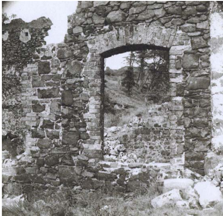
Figure 4.6 – Portion of the façade of the mill building, looking north-north-west (McC ANT 2712).
