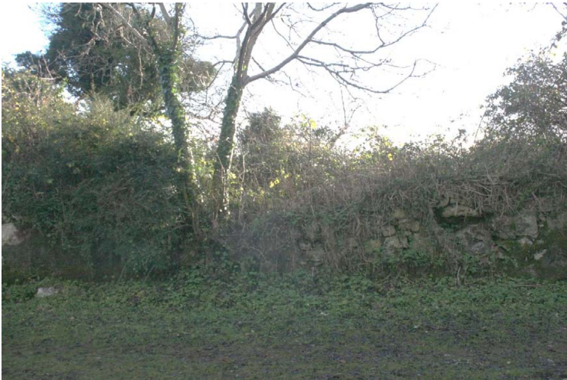
Figure 1.7 – North-western wall of building 'C', looking south-east.
