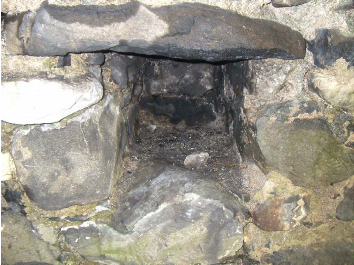
Figure 2.6 – Cavity within southern wall of the arched recess.
