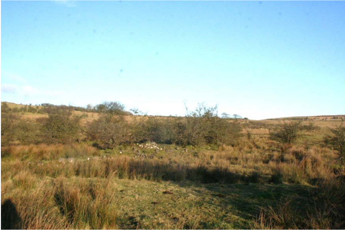
Figure12. 4 – The ruin is almost unrecognisable as a building, looking north-east.
