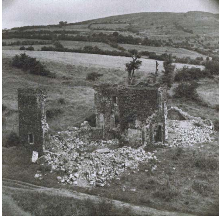
Figure 4.5 – The mill building and adjoining houses, looking north (McC ANT 2709).
