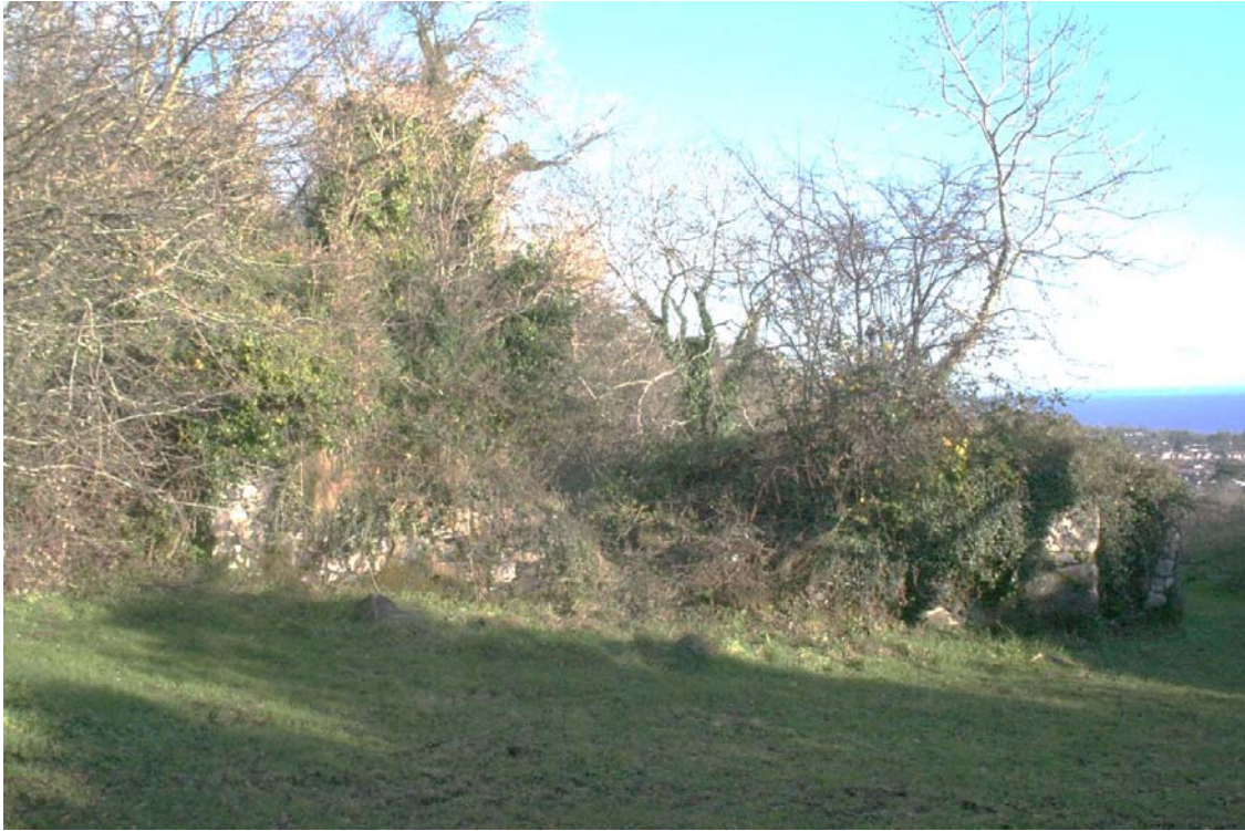
Figure 1.8 – Building 'B', south-western wall, looking north-east.
