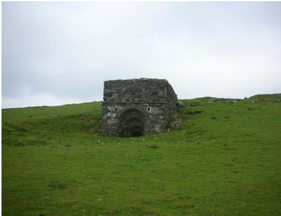
Figure 2.2 - Joist holes and ledge, above recess for fixing lean to against the lime kiln at Bighouse, Co. Antrim (after Welsh 2011, figure 6).
