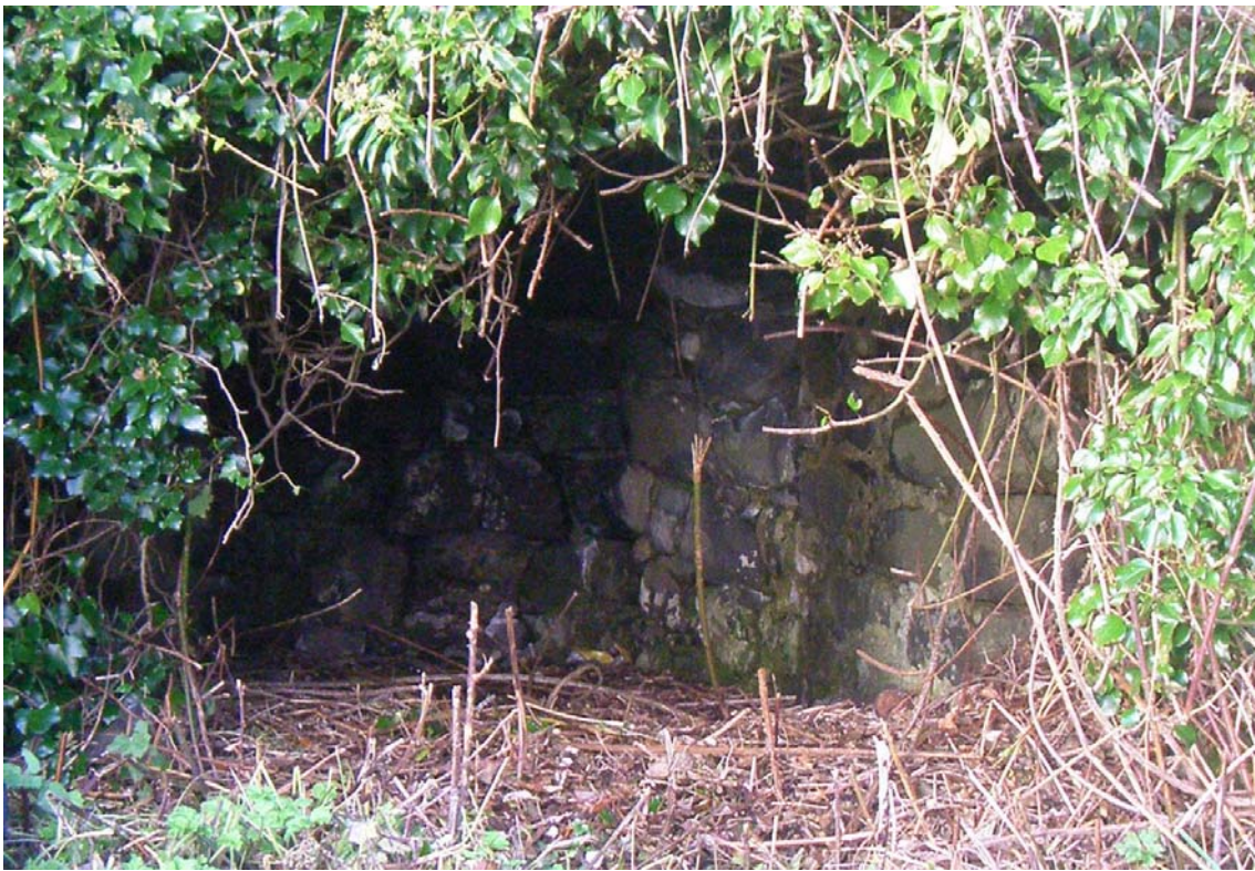
Figure 2.5 - Arched recess at Duanney lime kiln (IHR 1026500000).
