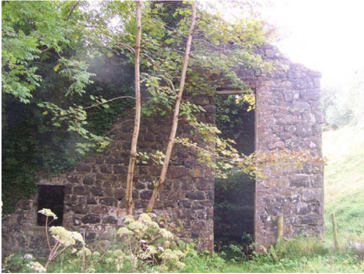
Figure 5.11 - Elongated ope in the northern gable of the 'corn mill'.
