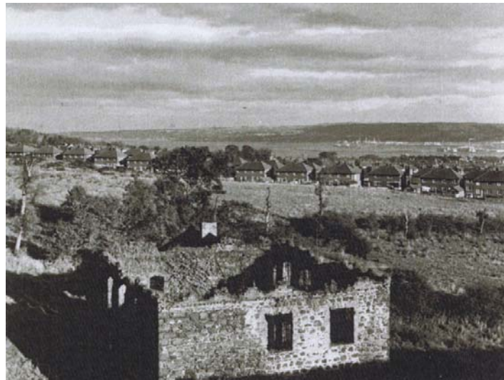
Figure 4.4 – The mill building and adjoining houses, looking east-south-east (McC ANT 2707).
