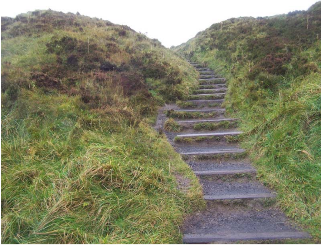
Figure 3.4 – Steps cut into the steep slopes.
